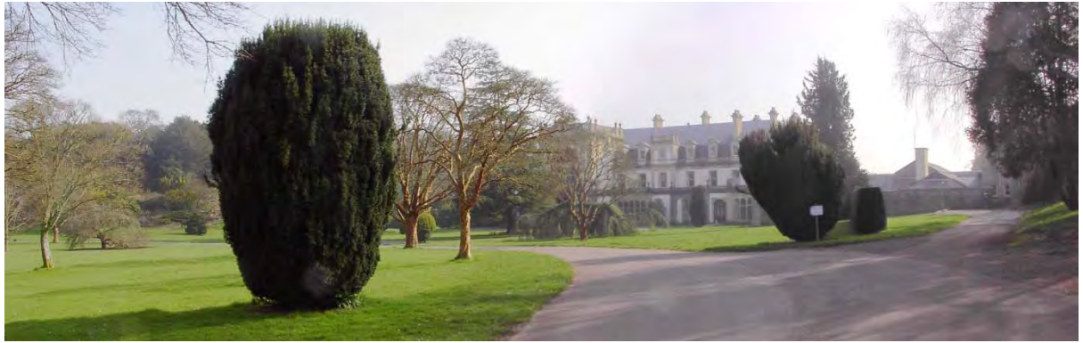
Existing view of the Dyffryn House as it is approached along the North Drive
