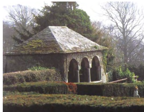
Edwardian pavilion built within the terraced gardens of St Donat's Castle
